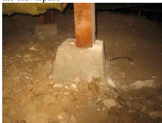
Sample view of a temporary pier & post installed
