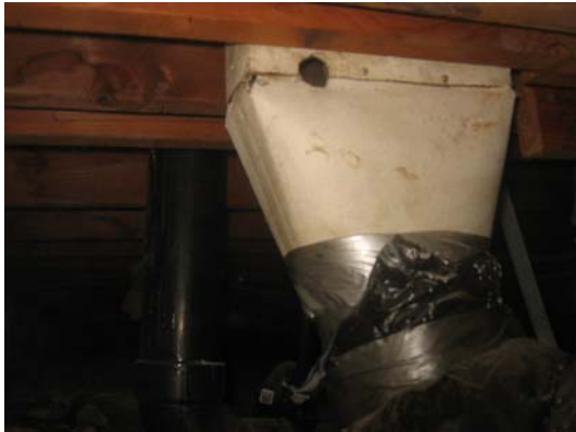
Sample view of materials that could possibly contain asbestos on the ducting
